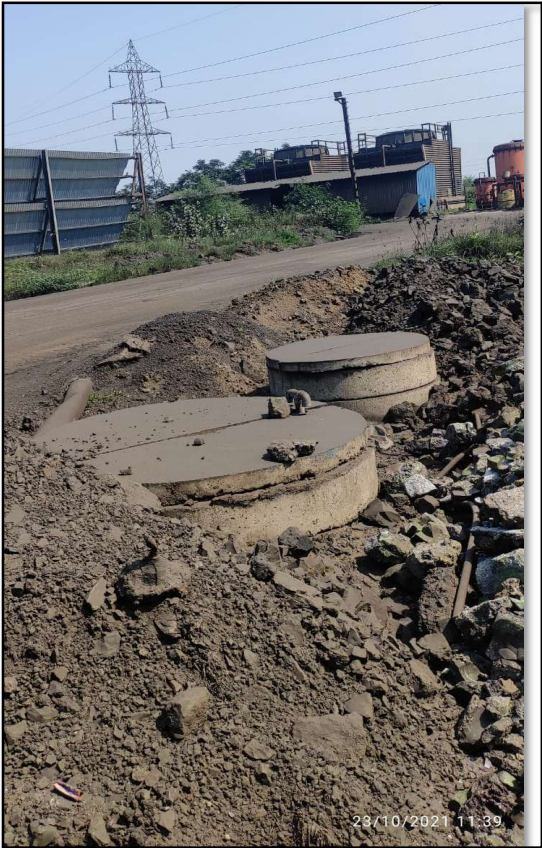
Pit No. 3 (Near ferro alloys unit)
