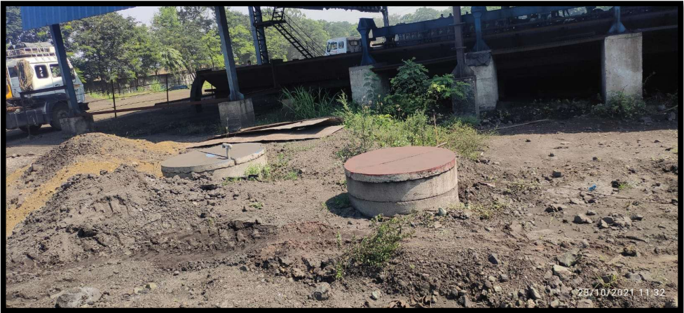
Pit No. 4 (Near Rolling Mill)
